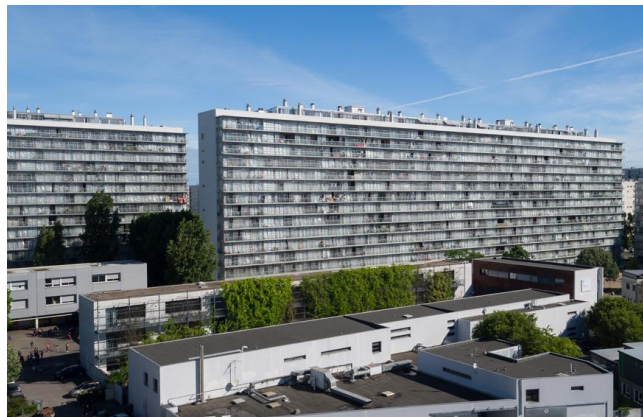
Transformation of G, H, I Buildings, Grand Parc, 530 Units, Social Housing (with Frédéric Druot and Christophe Hutin), photo courtesy of Philippe Ruault
